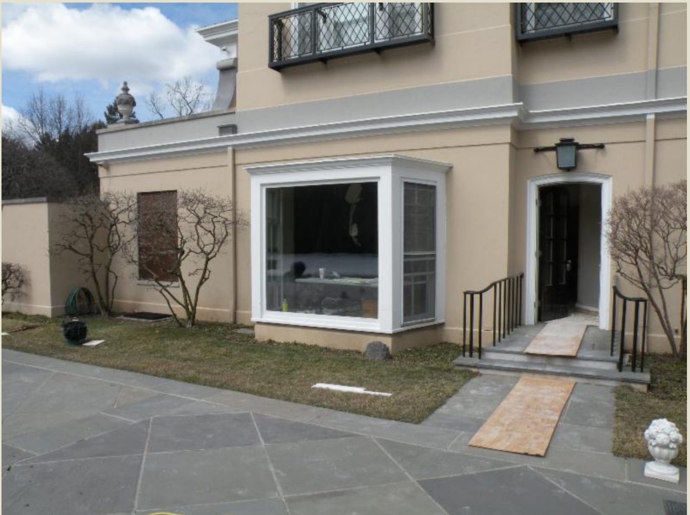
Before Picture - Demolition
