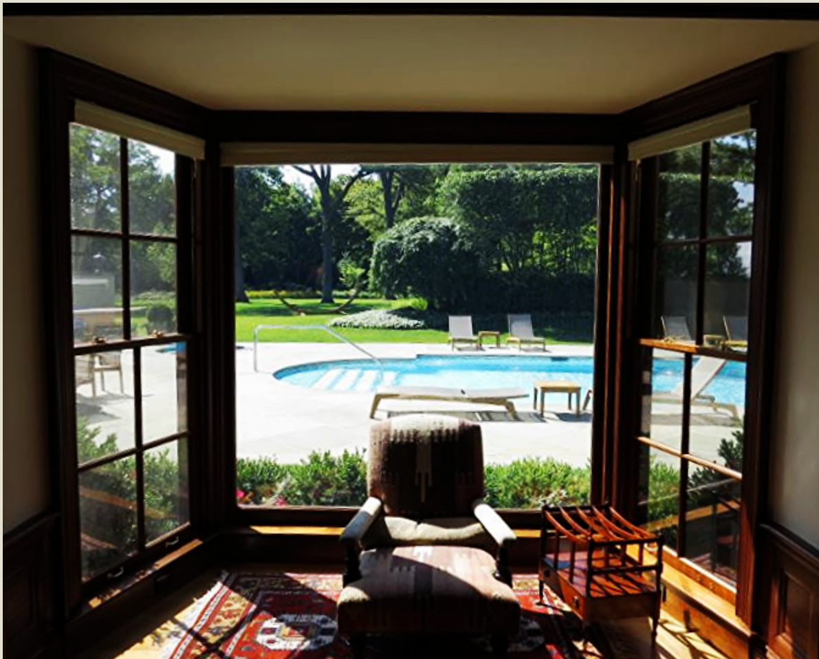
Bay Window - After Installation (Interior)
