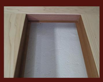
View from the interior side of the door. The location of the insulated glass which provides the look the customer wanted with the added benefit of energy-efficiency.
