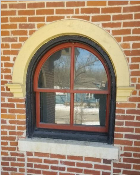
Before--Unprotected Primary Sash and Plexiglass Storms
