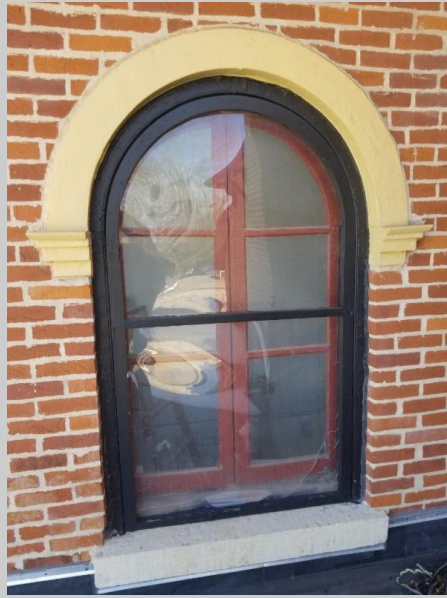
Before--Unprotected Primary Sash and Plexiglass Storms
