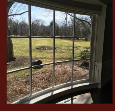
When the radius of the bowed sash is provided, we make a template to match. The wood is then carefully bent and glued up to obtain the necessary jamb depth. Once the exterior frame is completed, the muntins are added for each of the tru-divided lites.
