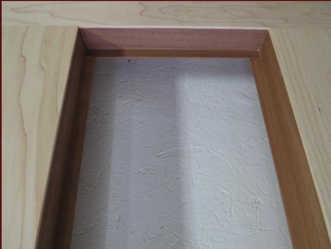
View from the interior side of the door. The location of the insulated glass which provides the look the customer wanted with the added benefit of energy-efficiency.
