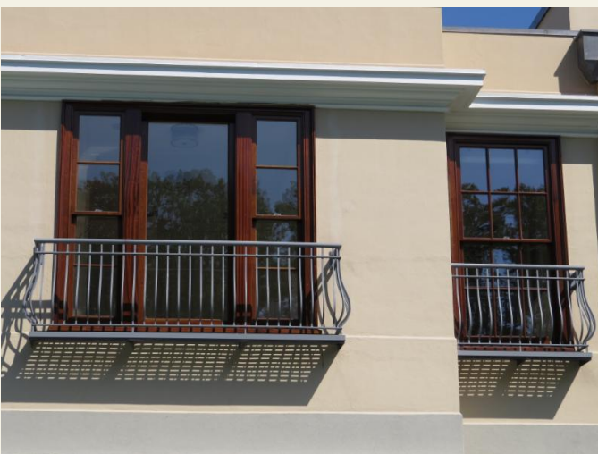
Second Floor Windows overlooking pool
