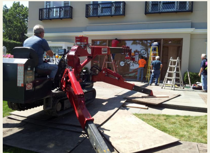
Installing the Glass into the sash Pictures Thanks to Jim Eimmerman, James LaDuke & Assoc.
