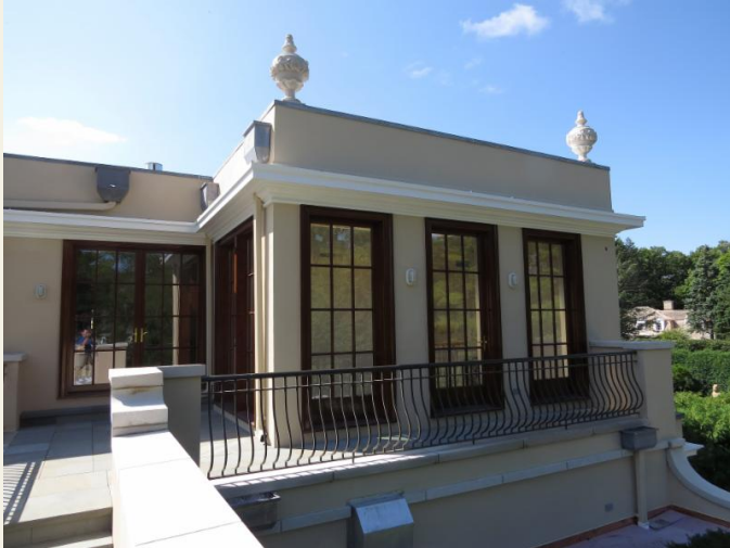
View of the doors leading to the deck area
