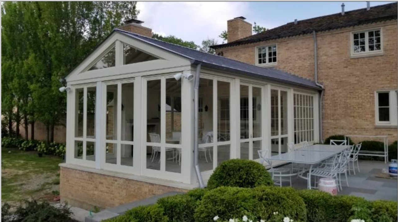
Closer view of completed three seasons porch addition
