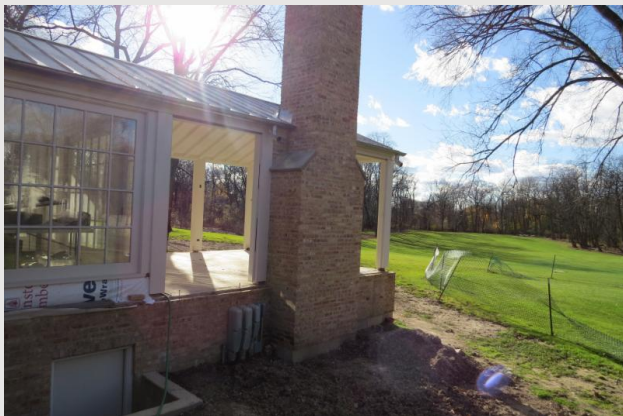
Mid-construction of the screened area.
