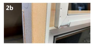
1. To remove the interior "moving" glass panel, you need to raise it up past the grey plastic piece that holds it in place. You can pull the bottom of the storm panel toward you.
