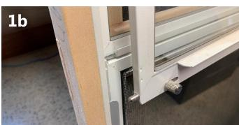
2. The next step is to remove the top "fixed" storm insert. To do this, you will need to lift the panel above its grey insert shelf and pull the bottom toward you (the top will be to the interior of the top metal piece that holds it in place.
