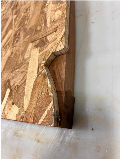
The project primarily revolved around replicating the historic windows of Brucemore, Templates were used to scribe the custom cut-out to ensure they maintained their original
