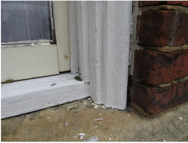
Picture of the original sill, frame, and brickmould.
