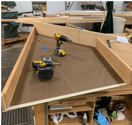
Window frame with brickmould, ready to attach custom sill.
