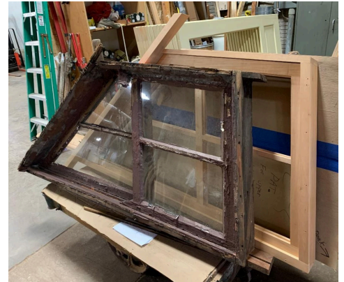
The existing sash is in front of the newly fabricated sash. Matching the angles was imperative for an exact fit.
