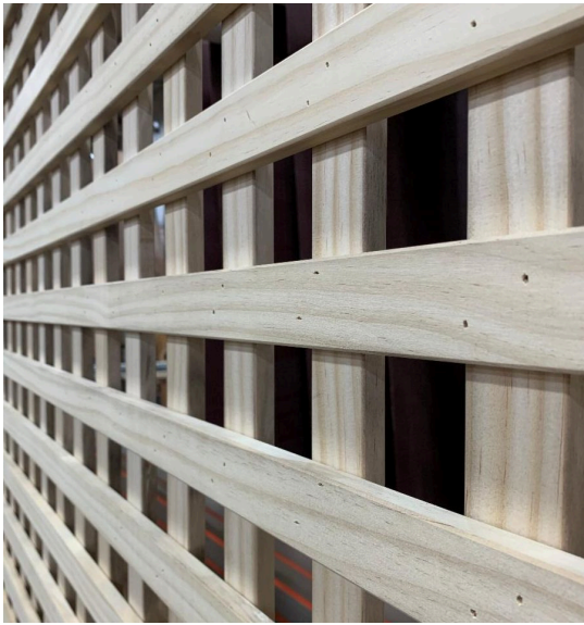
Trellis pieces measured 1-1/2" wide by 1/2" thick, forming 2" x 2" square spaces.
