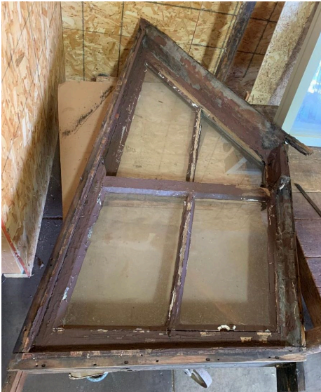
Original attic window sash.
