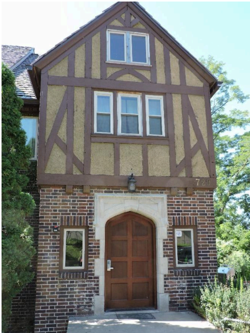
Installed new gothic top door.
