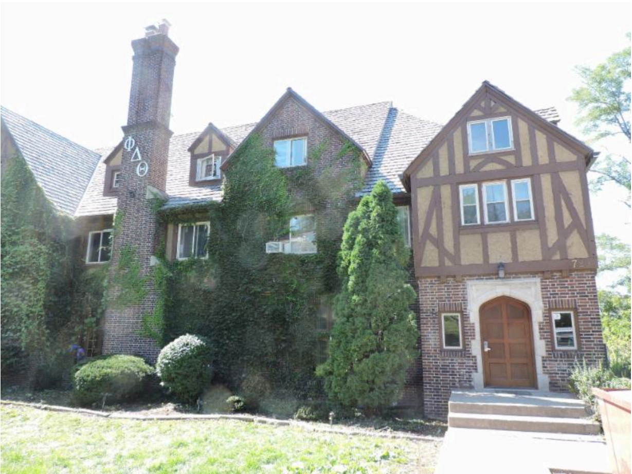
The new entry door installed.
