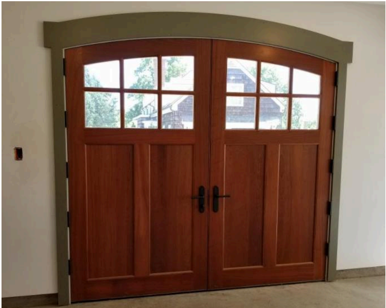
View from the interior of the Carriage House
