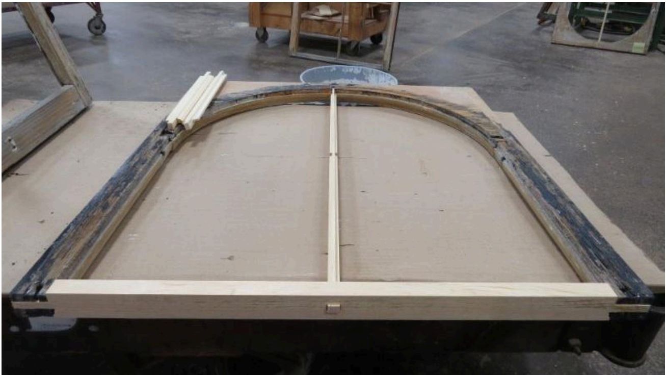
Working on replacing muntin bars and bottom rail in this sash.
