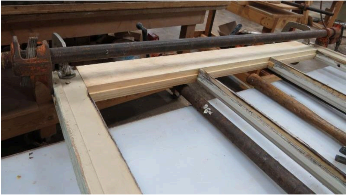
Picture showing another window sash getting a new bottom rail and being clamped.
