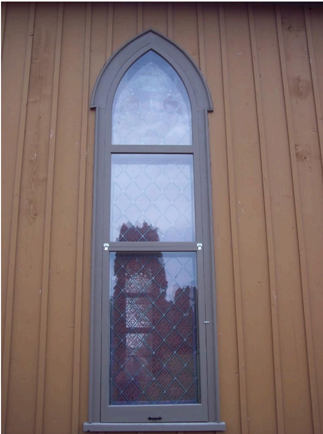
Gothic Top Installed
