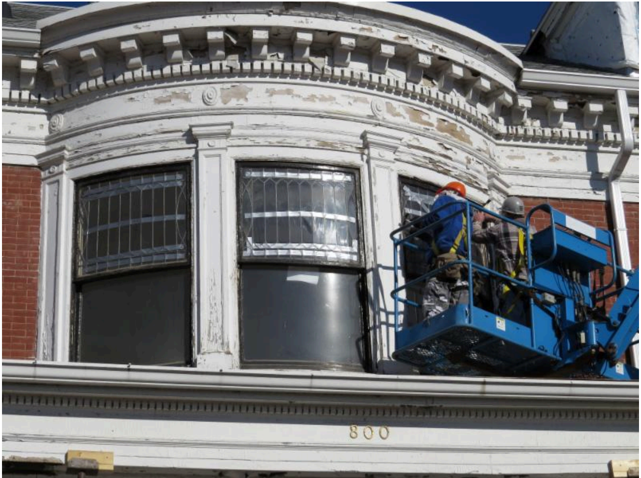
Measuring and taking out old windows
