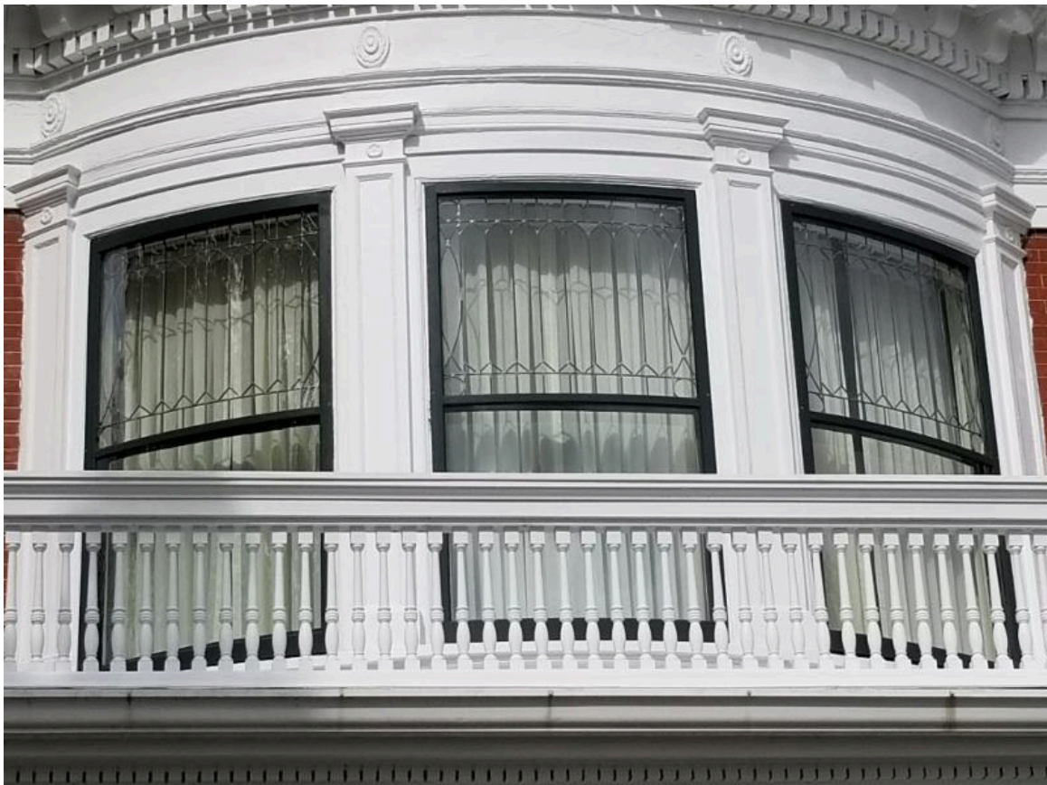
New storm windows in place
