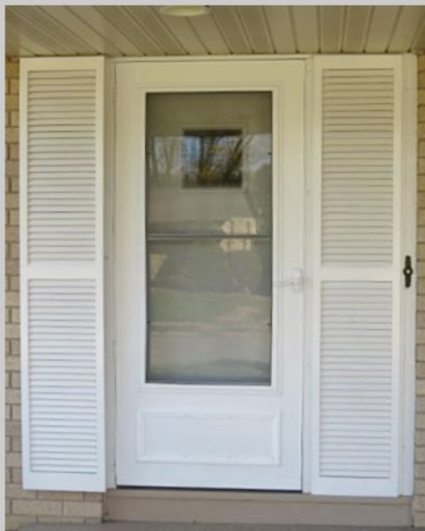
Original Entry Door
