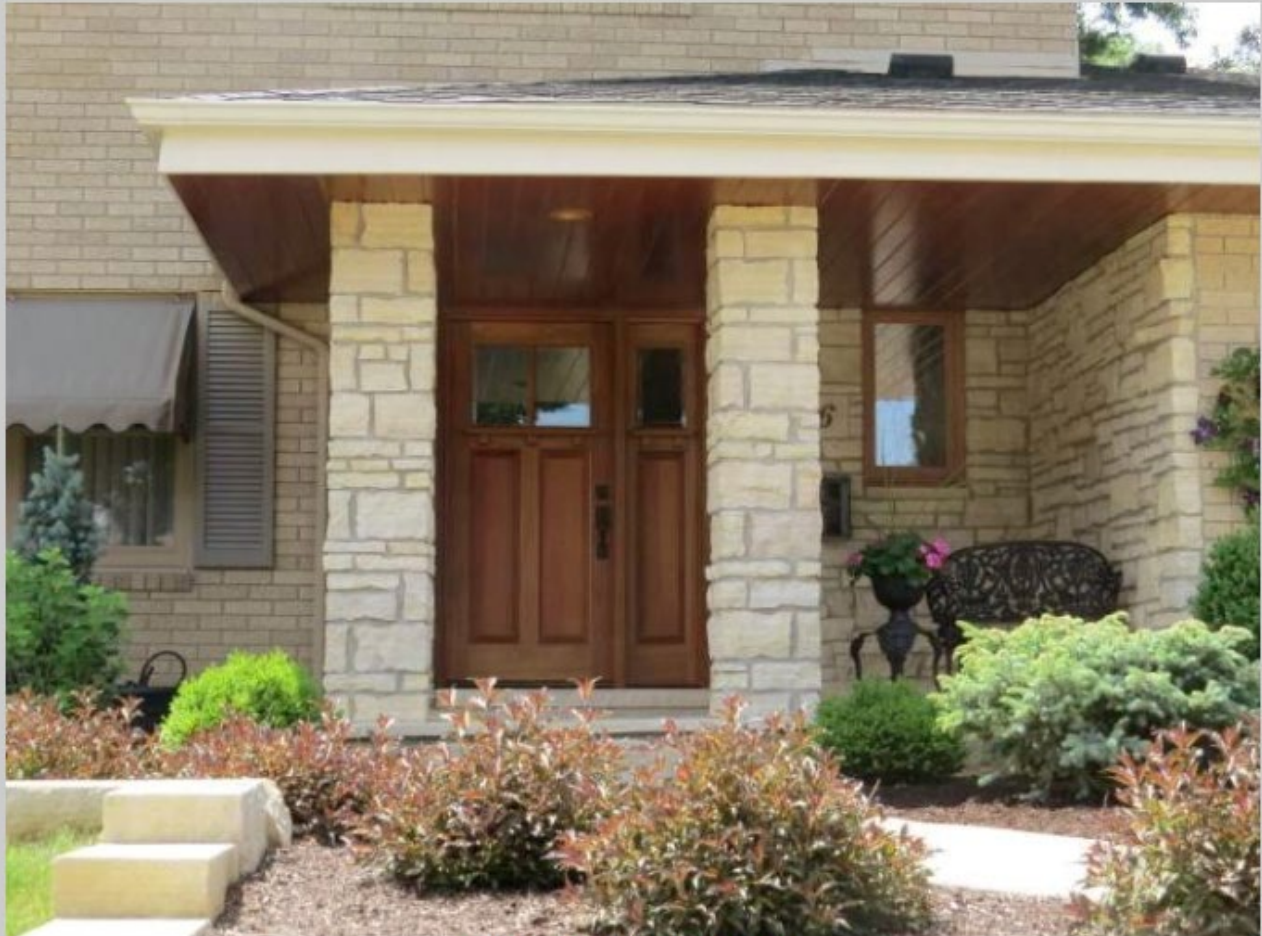
Completed Entryway Remodel
